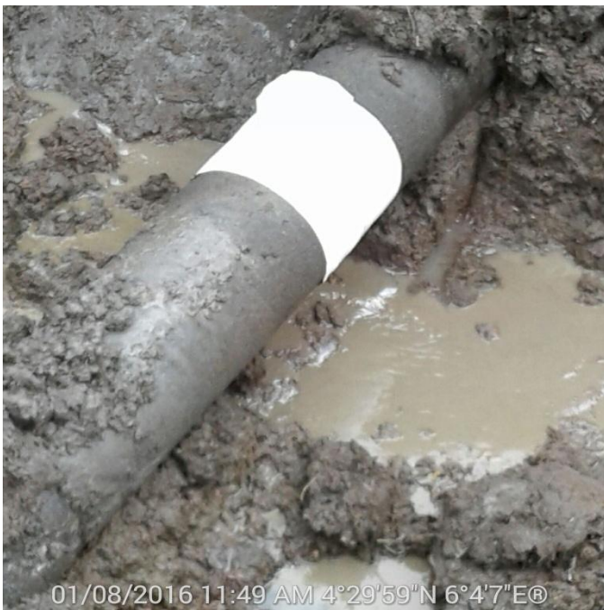
Fig C: Repair Work Completed
