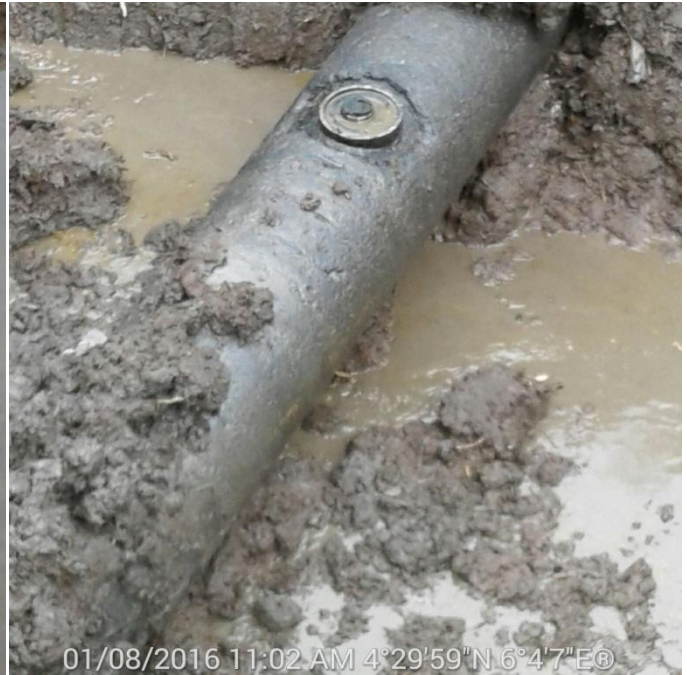
Fig B: Incident Facility after excavation
